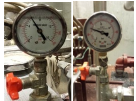
Inlet & Outlet Gauges measuring 6 Bars and 10.5 Bars respectively across the Oil Filter of the Yankee Unit Oil Filter
