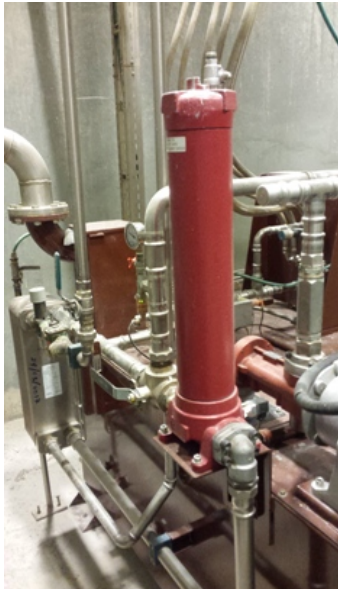
Yankee Unit of PM Oil Circulation
